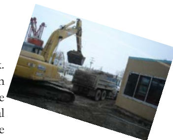
Expansion site of Okotoks Public Library
